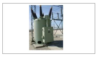
Fig. 4.1.19 Oil Circuit Breake
